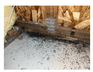
Moisture stains were found over the master bedroom to truesses and ceilings. The source of the moisture stains appears to have been a leak at the rear master bedroom wall and ceiling where wood rot was found.
